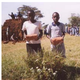
Bricks were made locally for the construction of the classrooms
